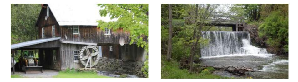
Well-preserved remains of a class 3 mill system in Van Hornesville (see also below). Notice that the waterwheel remains on site (left), and the dam upstream is well-preserved as well. The race itself, however, is absent.
