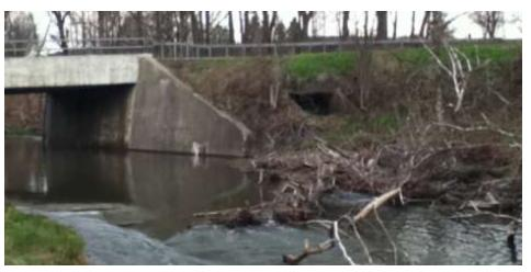
Downstream side of North Street Bridge, Hartwick. Notice tunnel at right of bridge for race.
